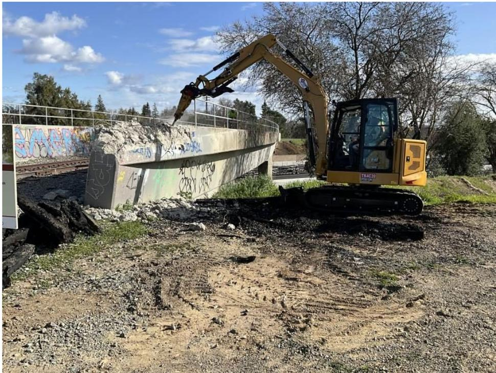
Crews are demolishing a portion of the wingwalls of the existing Land Park Underpass Bridge to prepare to widen the bridge overhang as part of the new trail alignment over I-5.
